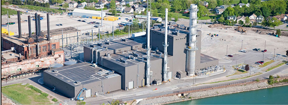
Thorold Cogeneration Station
